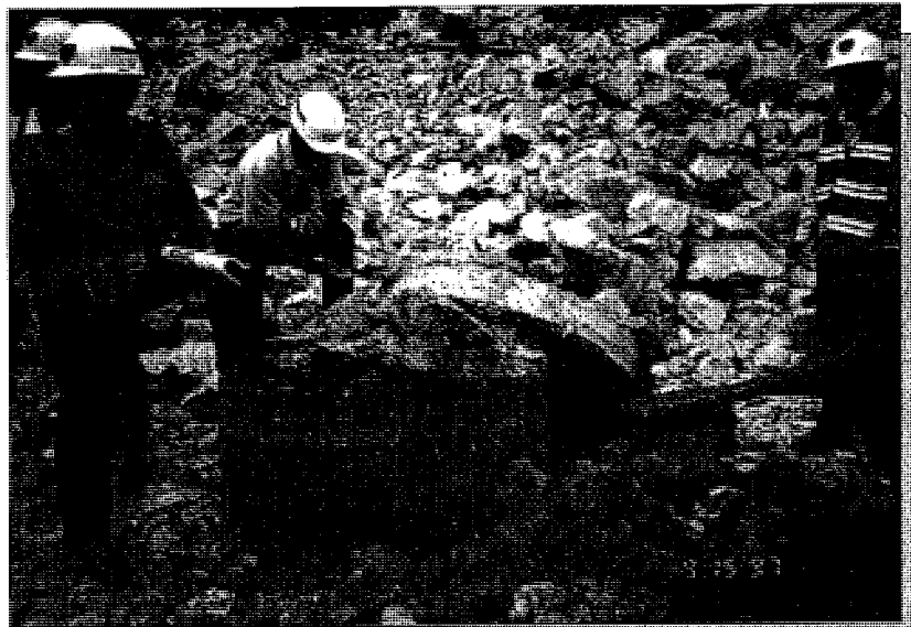
Construction workers are shown in this photo working on the foundation for Pier No. 1. The bridge contractor, Mark Blum, Inc., is shown in this photo working on the foundation for Pier No. 2. The bridge contractor, Mark Blum, Inc., is shown in this photo working on the foundation for Pier No. 3. The bridge contractor, Mark Blum, Inc., is shown in this photo working on the foundation for Pier No. 4. The bridge contractor, Mark Blum, Inc., is shown in this photo working on the foundation for Pier No. 5. The bridge contractor, Mark Blum, Inc., is shown in this photo working on the foundation for Pier No. 6.
